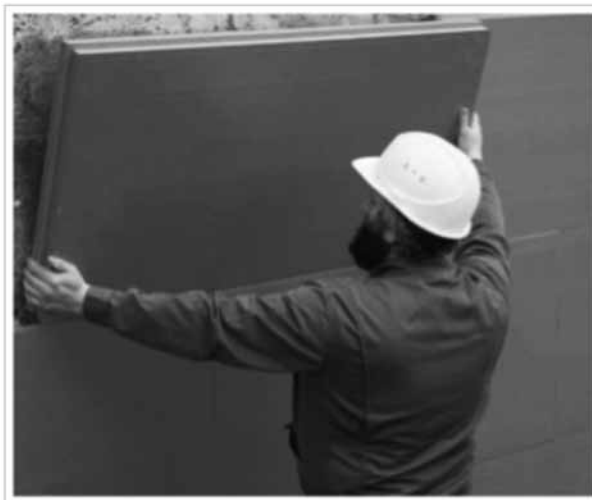
Figure 11. Application of XPS insulation boards on a basement wall
